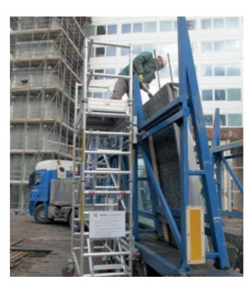
The hanging rolling scaffold makes it easier and safer to unload vehicles without using a ladder.
