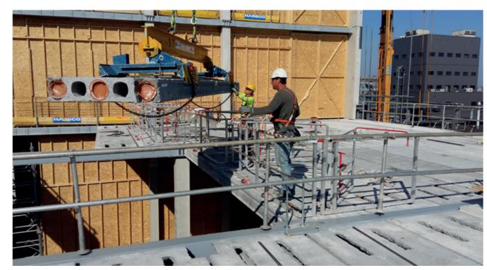
The first application of the belt-free system, developed in-house, for the safe installation of hollow core slabs.
