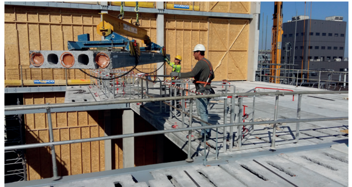
The first application of the belt-free system, developed in-house, for the safe installation of hollow core slabs.
